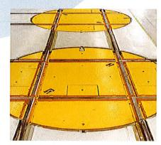
**Turntables** are extremely rugged and well-balanced and are used to rotate bogey trucks to allow them to be transferred to other tracks.
