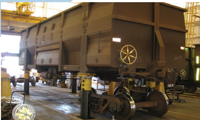
Hydraulic Repair in Place (RIP) Jacks facilitate the quick repair of railcars to return them to the main line.
