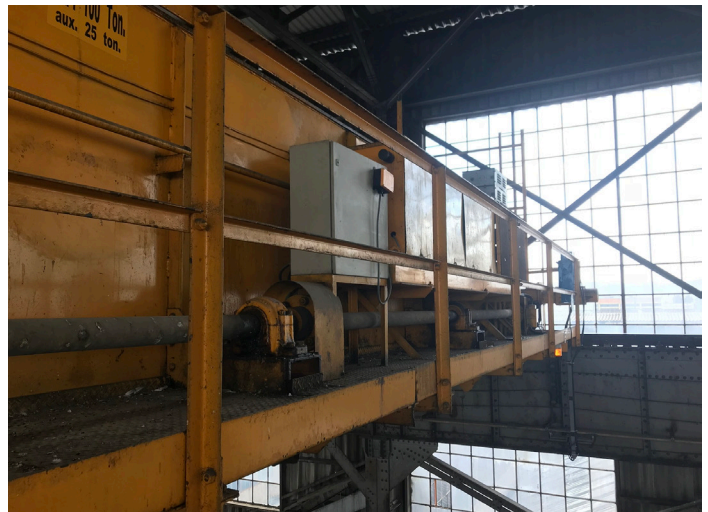
Damaged and improperly installed controls before modernization
