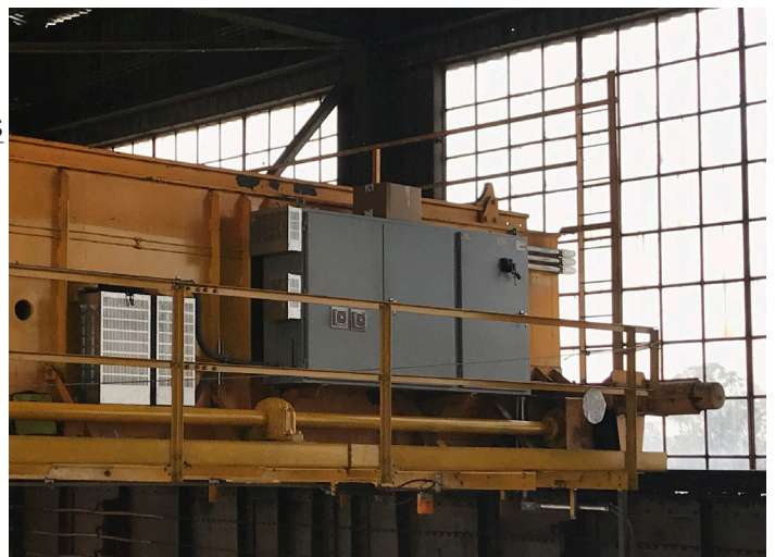
Controls after modernization
