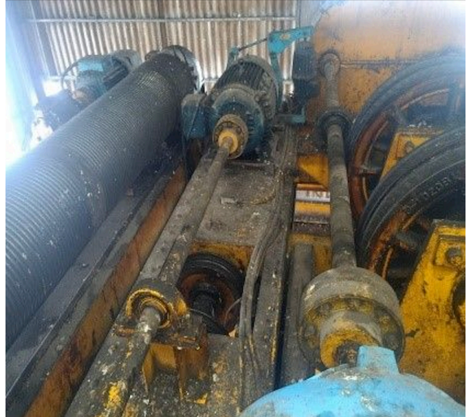
Trolley deck before modernization
