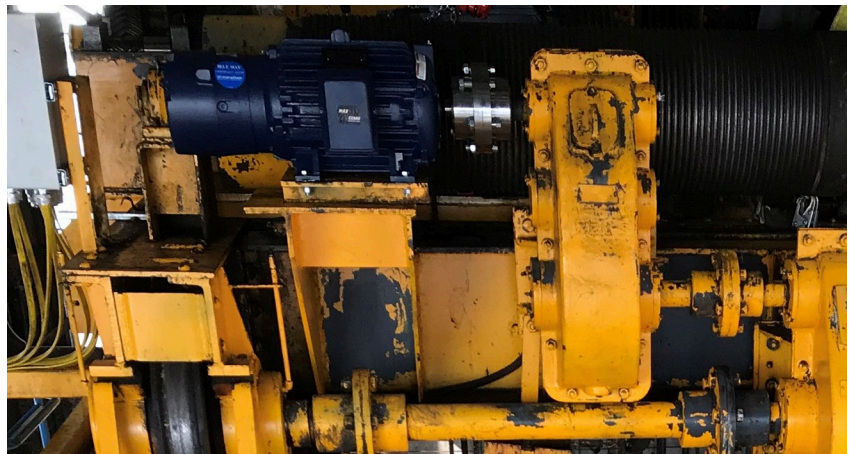
New trolley deck after modernization
